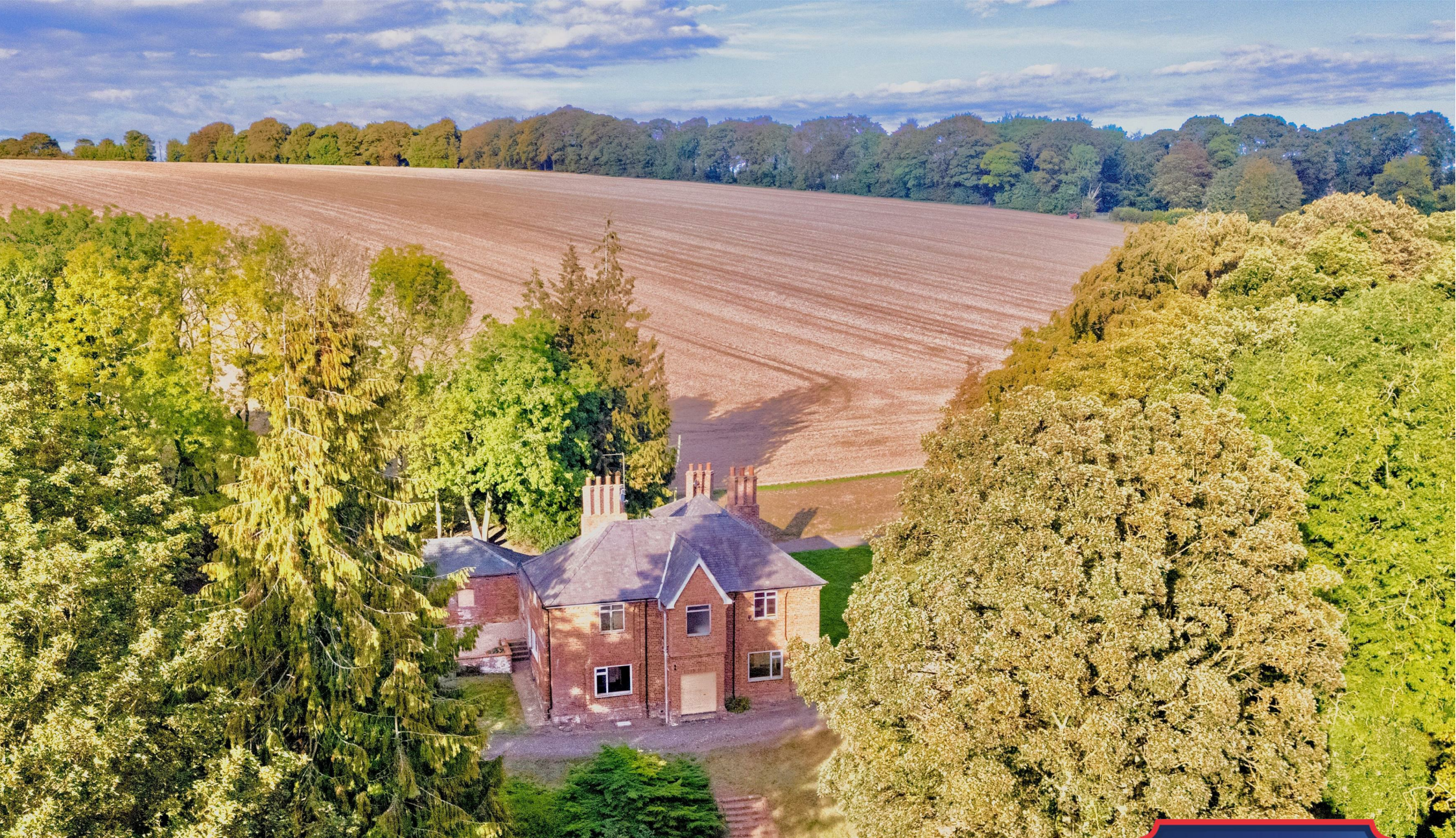
The Rectory, Ruckland Louth, LN11 8RQ
